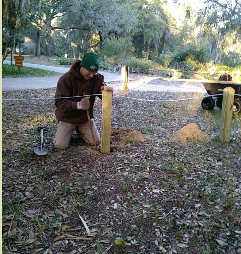
Volunteer Alex Wolf helps with the installation of new, solid wood stakes and protective wire around the large oak at the entrance of the Jacksonville Arboretum & Gardens.
